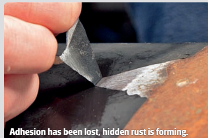
Adhesion has been lost, hidden rust is forming.
